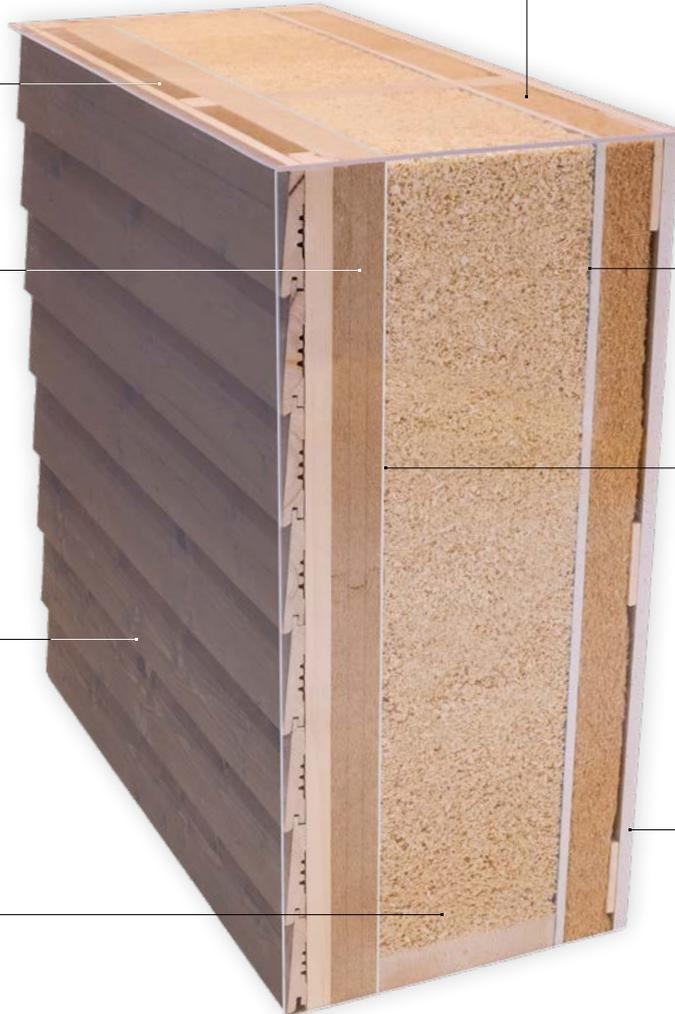
The 46cm-thick Baufritz AAA wall achieves thermal insulation values of a low as  $0.13\text{W/m}^2\cdot\text{K}$
