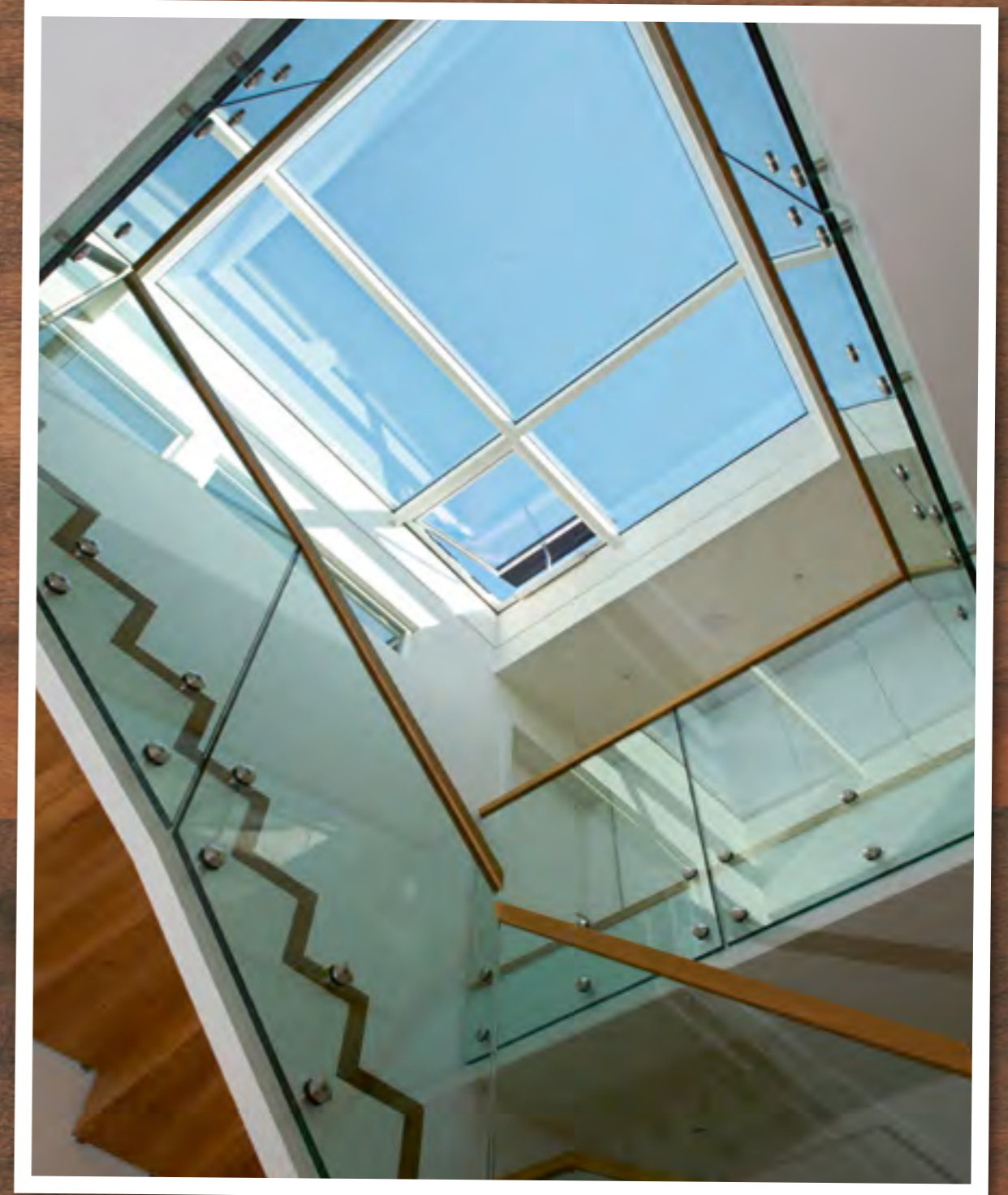
With a size of nearly 10 m 2 , the skylight floods the core of the house with natural light.
